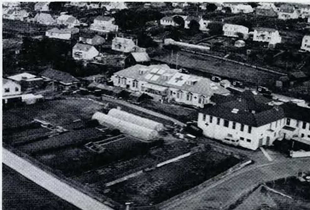
Fig. 1. King Edward Memorial Hospital, BMH, Falklands
